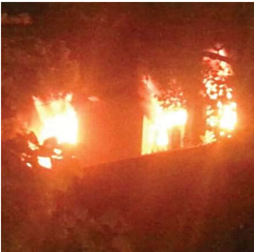
The IC&SR building of IIT Madras on fire on Wednesday night
